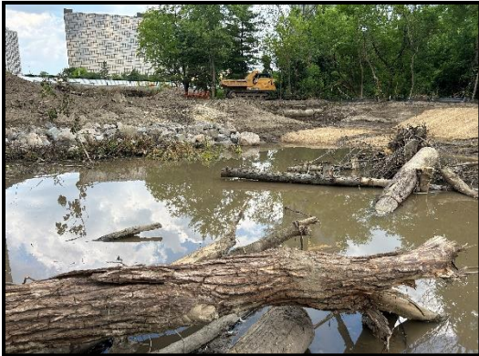
June 5, 2023 Habitat structures - north area
