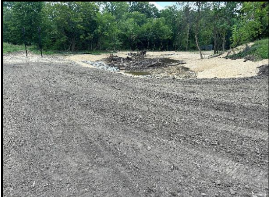
July 21, 2023 Site graded with erosion control in place
