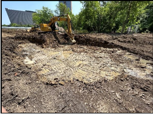
June 21, 2023 Wetland cell excavation
